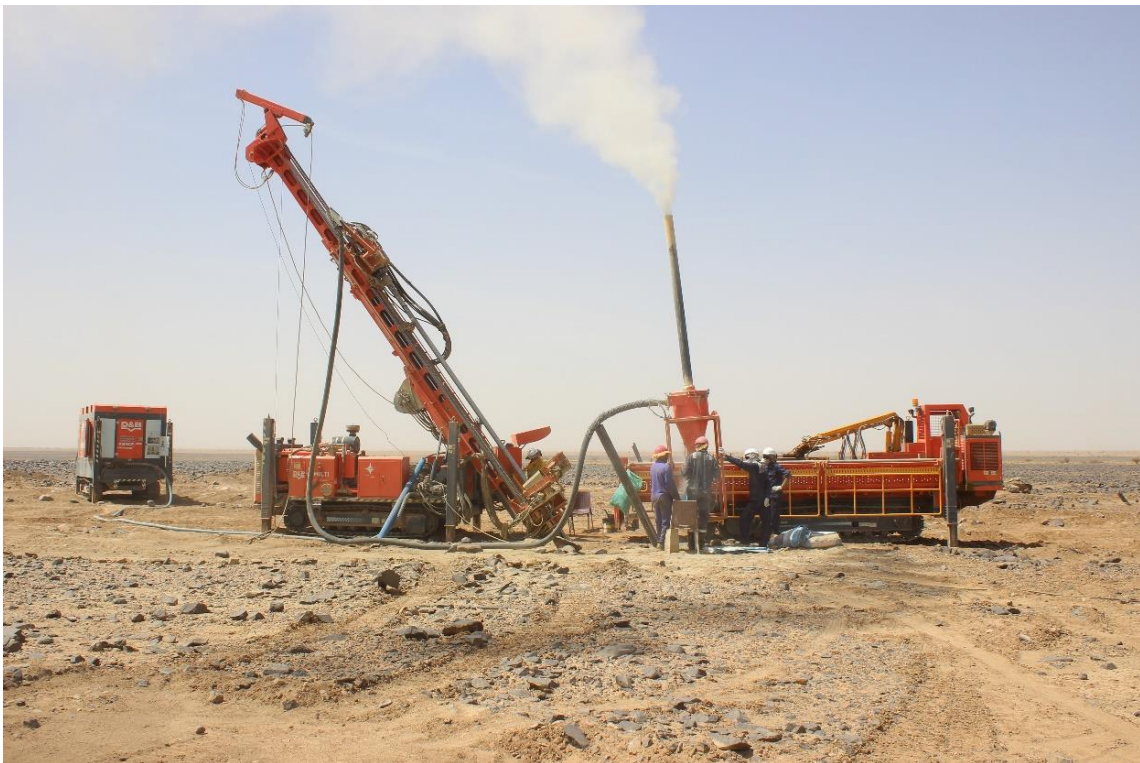
Fig 10.1. Drilling an inclined RC hole by D&B30multi rig.
